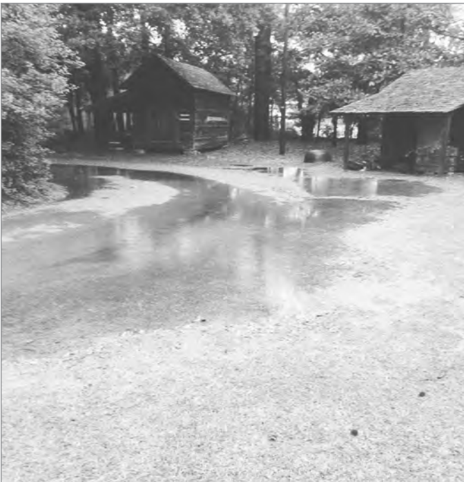
Water-logged grounds following heavy rain.
