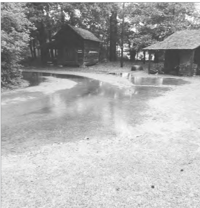
Water-logged grounds following heavy rain.
