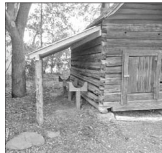
New lean-to attached to the corn crib. The addition will help protect the 19th century Pee Dee Indian dugout canoe.
