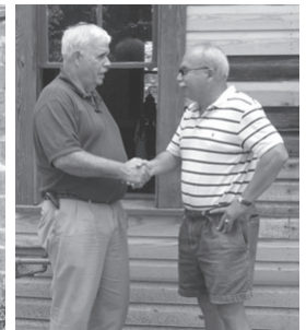
Zywocinski, right, shakes hands with Chandler upon completion of the Shaw House repairs.
